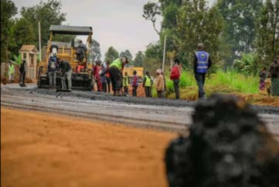
ROAD CONSTRUCTION UNDERWAY
