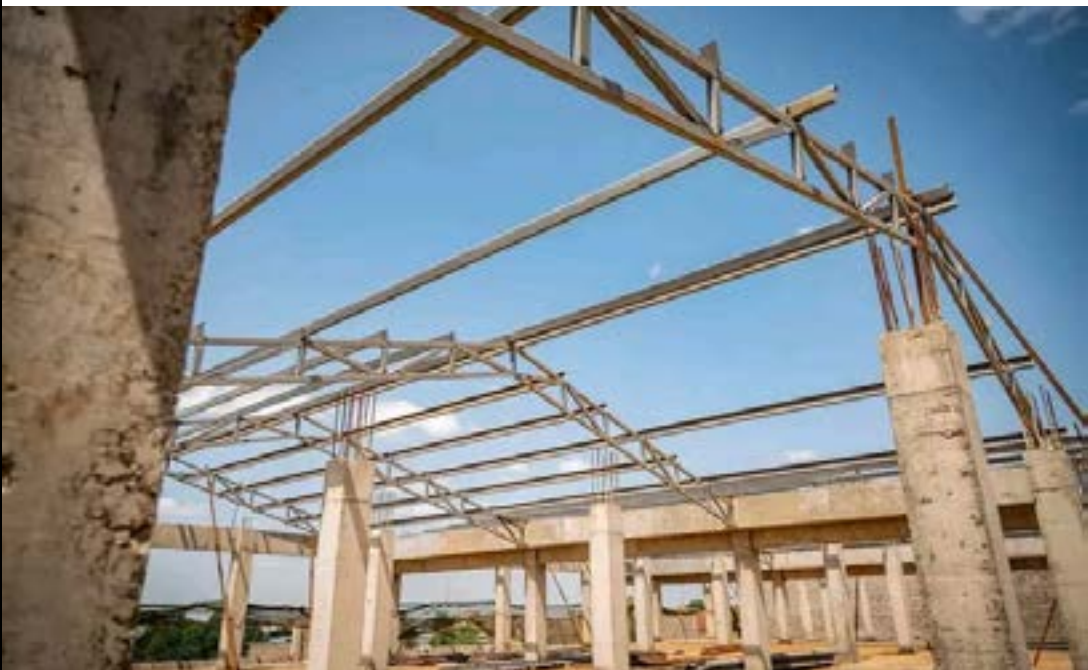
SITE CONSTRUCTION OF THE MODERN MARKET
