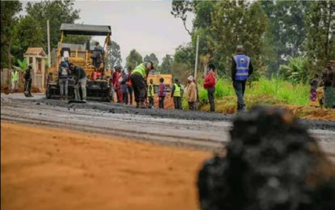
ROAD UPGRADE REMAINS OUR PRIORITY
